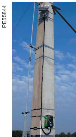
Solar panel for G2GF
